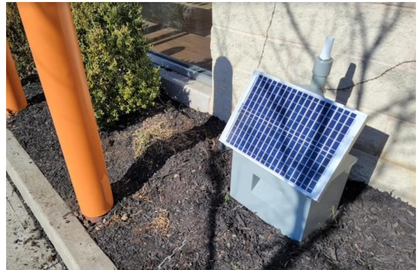
Remote Vibration Monitoring Station
